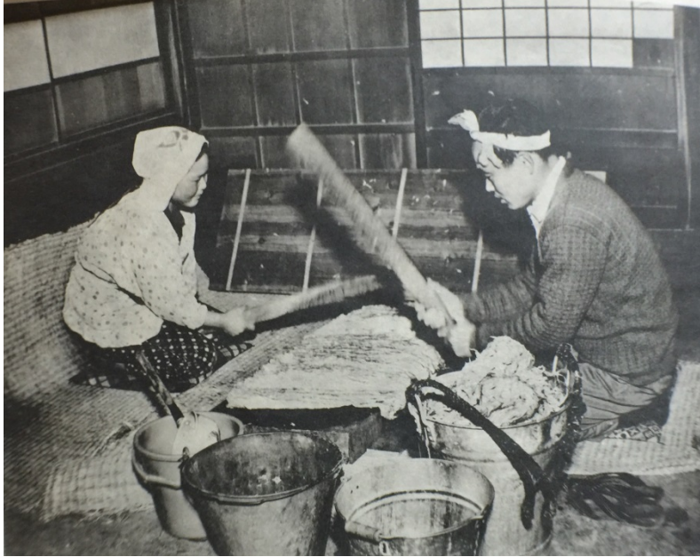
Figure 29 – Kurotani, Ayabe City. A husband and wife using wooden clubs to beat the fibers for papermaking.
